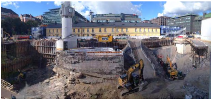
Excavation of Lasipalatsi plaza to accommodate subterranean Amos Rex art galleries and art storage space. Approximately 14,000 m 3 of soil and bedrock were removed.
